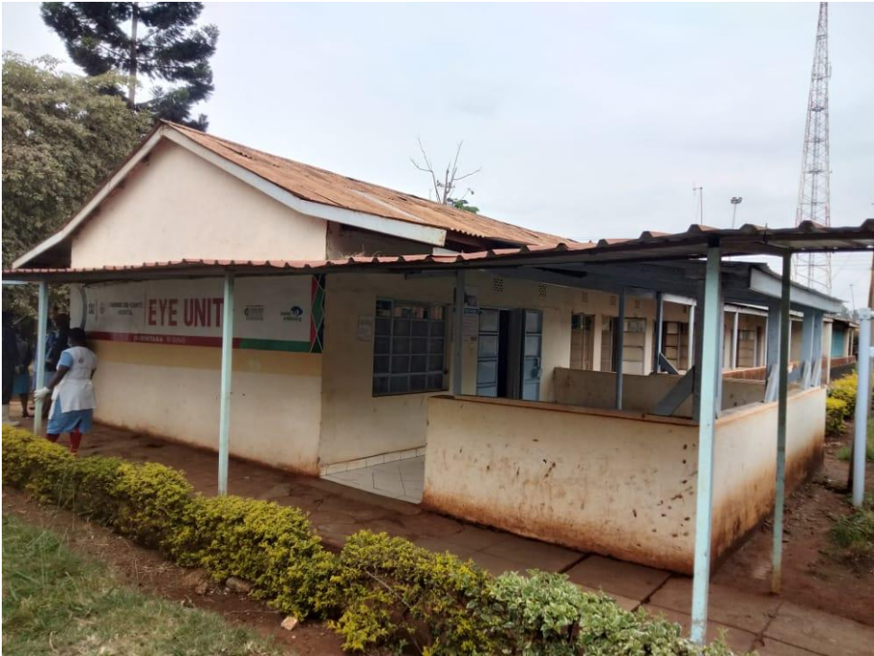
Newly renovated Kimbimbi Sub-County Eye Unit
